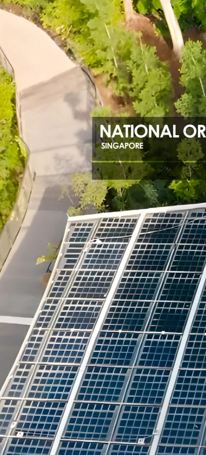
"The Cool House is designed to emulate a high elevation forest, which exists at altitudes of 1.000m to 2.000m, and with a surrounding temperature of 16°C to 23°C. Having in mind the extreme weather conditions of Singapore the selection of high performance glass with optimal passive properties was decisive."
