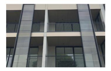
"The architecture takes full advantage of its corner address. Onyx Solar photovoltaic glass on the façade, is both a feature & practical. Optimizing the building orientation, the glazing absorbs light to power the building."
